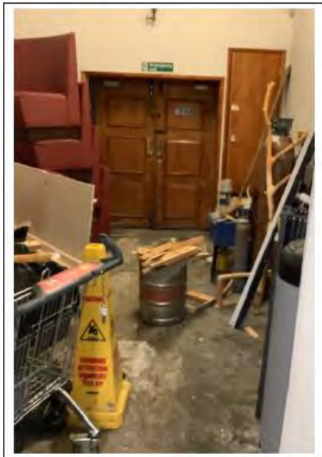
Obstructed fire exit and unsecured gas cylinders 18.1.23
