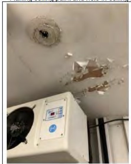
Flaking ceiling paint and hole in ceiling in cellar
